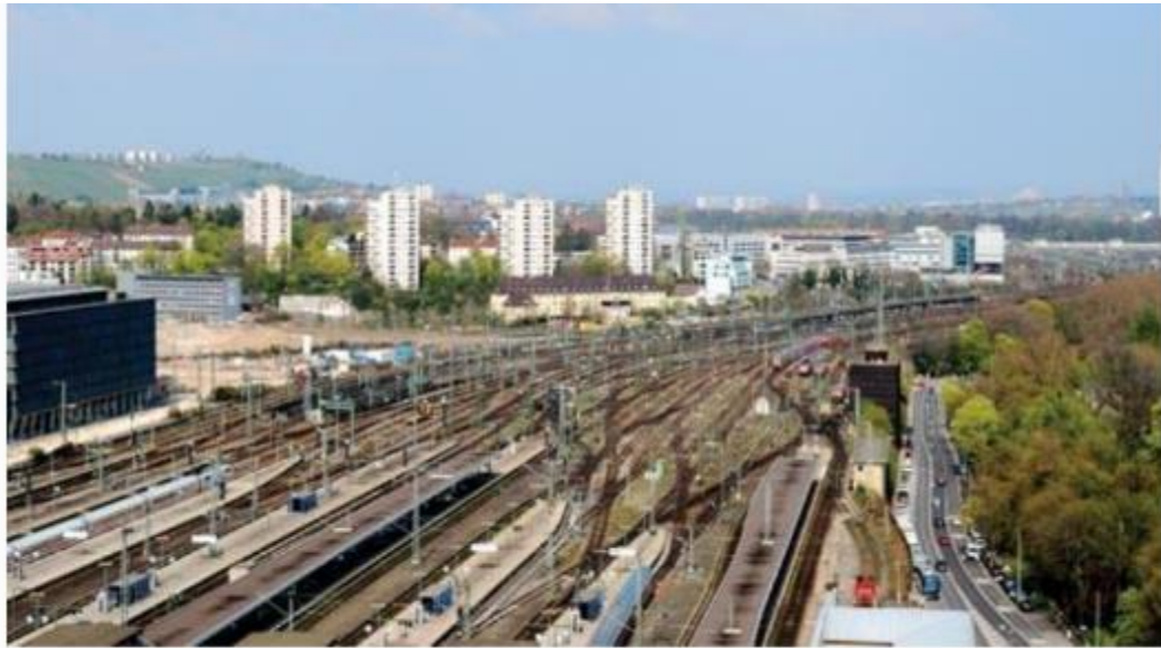
Stuttgart's main railway station.
